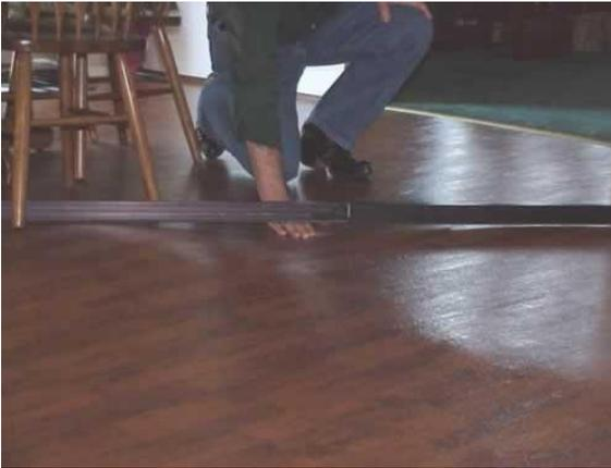
3. Cabinets should not be installed on top of a floating floor – For some reason, people want the flooring in first, and then they want the cabinets and islands installed on top of the flooring. This cannot happen with a floating floor. You have just locked this floor down and created a massive pinch point and sometime soon they will have a buckle in the flooring.
